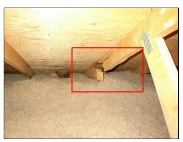
5. Top chord of truss is broken
