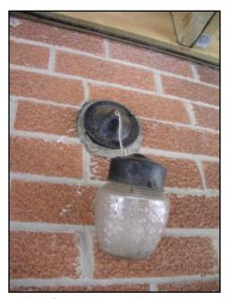
7. Light fixture is not well secured
