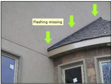
1. No kickout flashing at roof/sidewall junction
