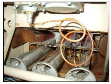
9. Rust at bottom of heat exchanger
