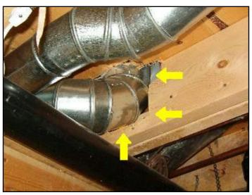
4. Double joist cut for ductwork
