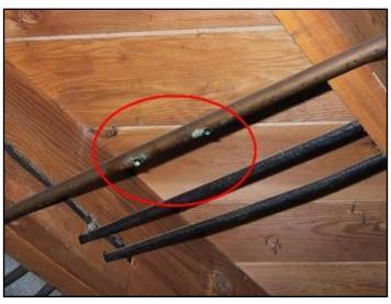
14. Leaking copper supply pipe
