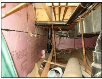
13. Exposed polystyrene insulation is fire hazard
