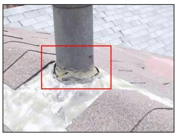
2. Stack flashing should be sealed.
